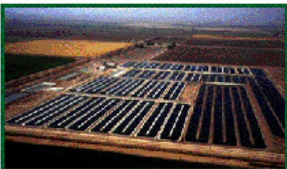
Earthrise Farms USA
